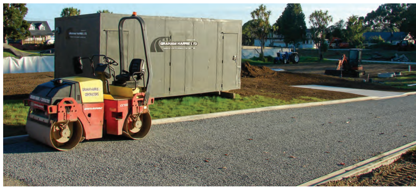
One view showing newly laid bitumen roading.
